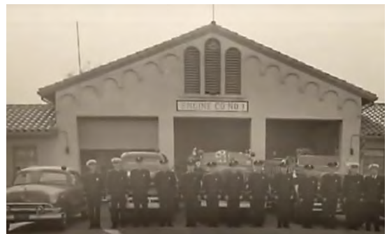
Figure CR-41. Colton Fire Station built in 1936 with WPA assistance. Source: Dennis Bickers, 2009
