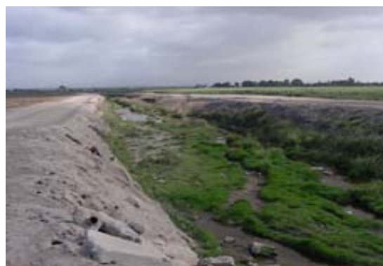
Figure 5-25. Unlined Open Channel Segment of Cypress Channel
