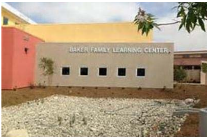
Figure 5-31. 1,760 Cubic Foot Basin Feature Located at the Front of the Learning Center
