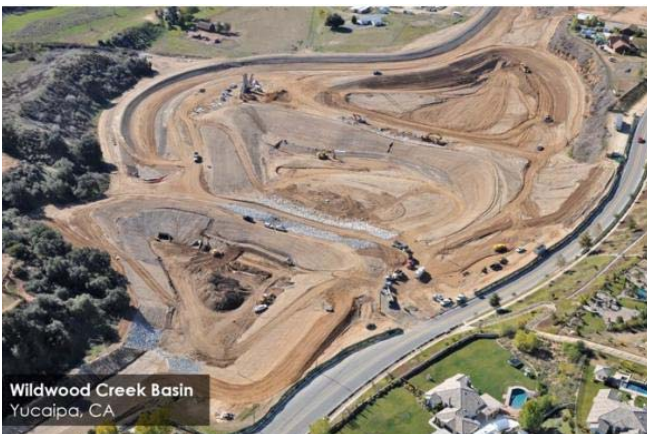
Figure 5-29. Construction of the Wildwood Creek Basin Project
