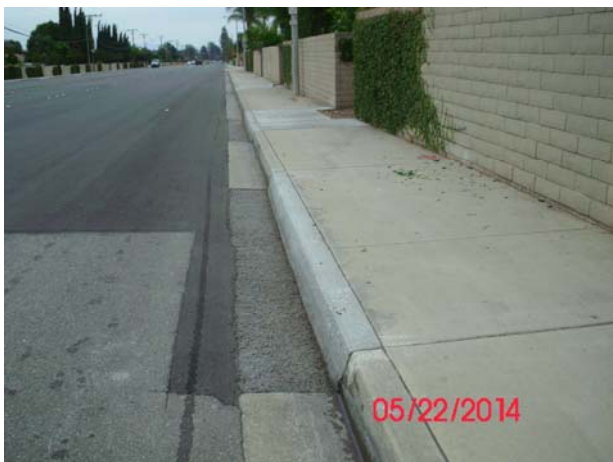
Figure 5-17. Installation of Pervious Concrete in Gutters on Ramona Avenue
