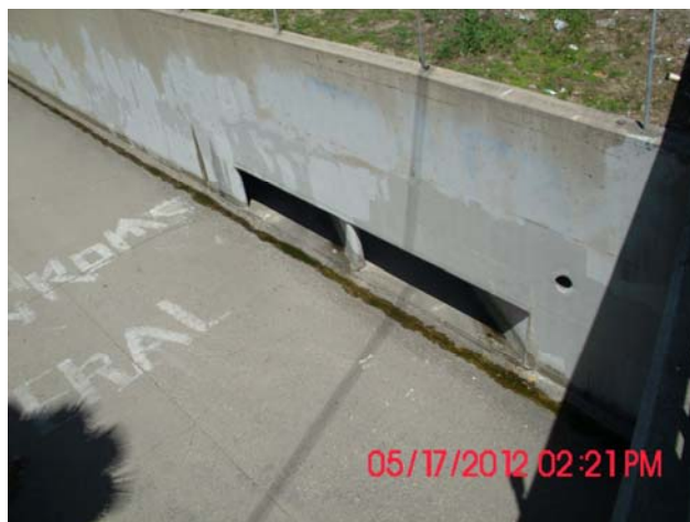
Figure 5-16. Lack of Dry Weather Flow from San Antonio Channel MS4 Outfall
