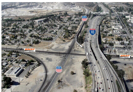
The Colton Crossing, prior to construction of improvements to construct the UPRR fly-over of the UPRR line.
